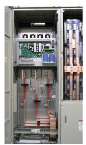
Rear of Interface Panel – Motor Connections at Bottom
