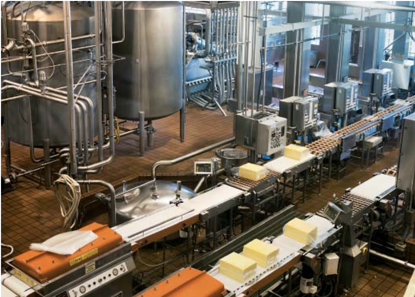
Manufacturing should be an integrated process; Mitsubishi Electric helps to achieve that goal
